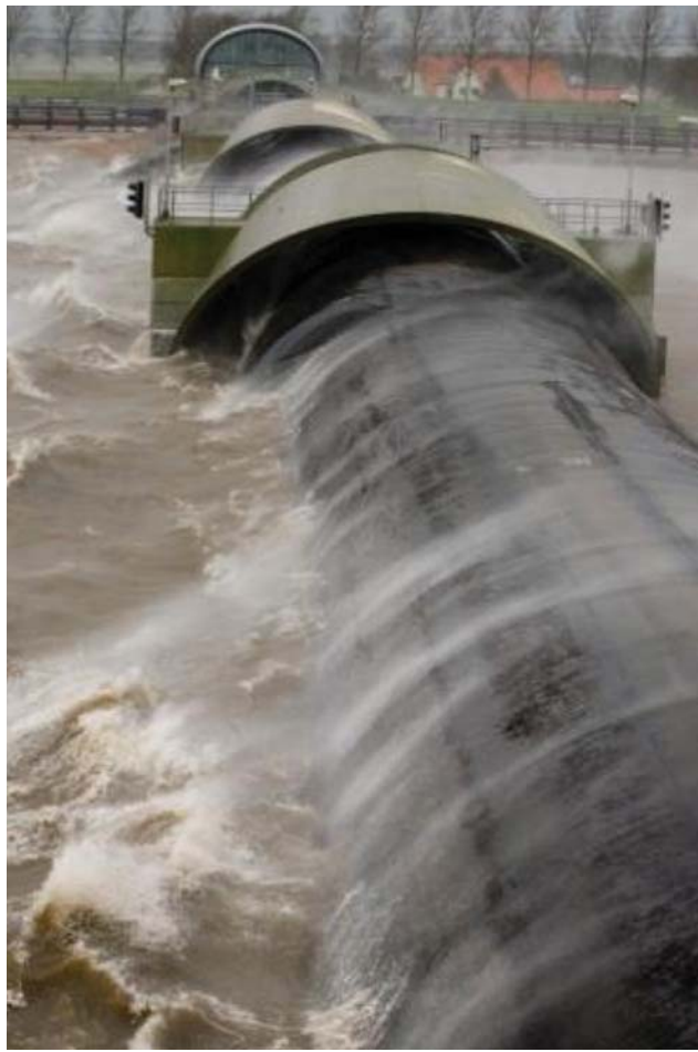
Figure 7-11 Inflatable Rubber Weirs at the Ramspol Storm Surge Barrier
