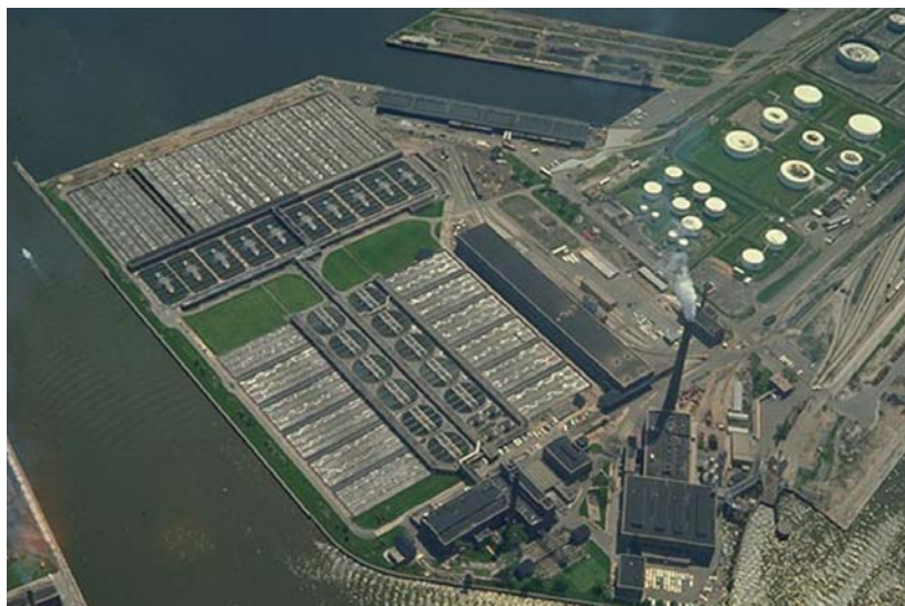
Figure 3-3 Wastewater Treatment Plant – Milwaukee, WI
