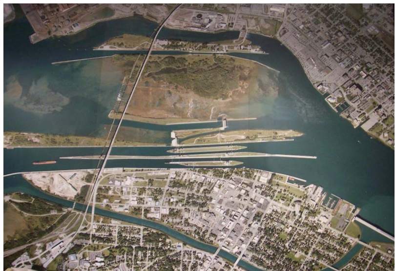
Figure 1-1 Lake Superior Regulation Control Structures
