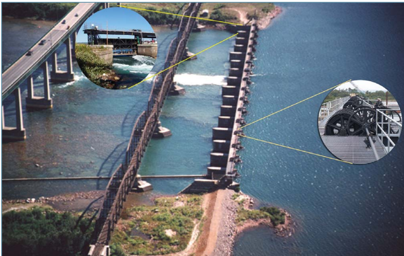
Figure 5-1 Compensating Works on the St. Marys River
