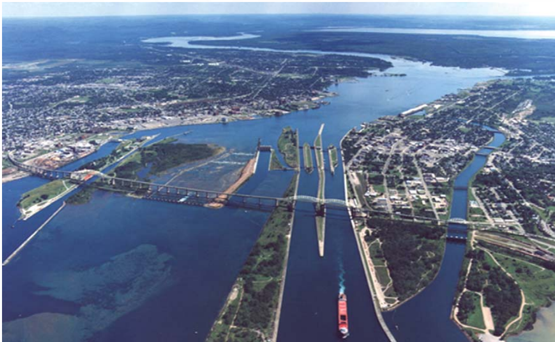
Figure 11-1 Lake Superior Regulation Control Structures
