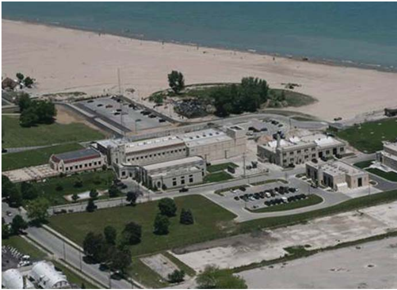
Figure 3-2 Water Treatment Plant – Racine, WI
