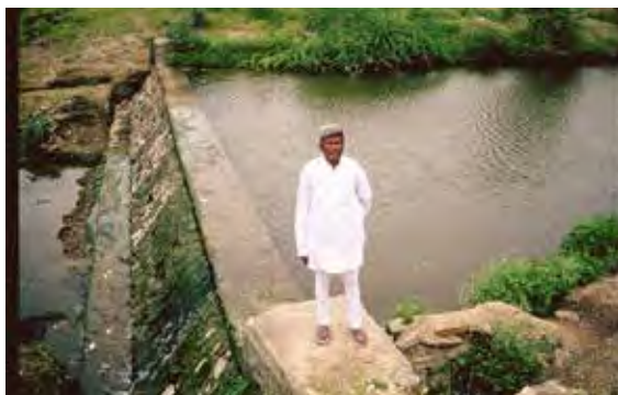
Man stands next to a johad, or small dam, built to impound rainwater in India. Photo: Patrick McCully
