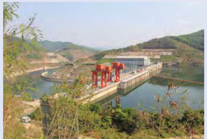
The 1,750 MW Jinghong Dam on the Lancang River was completed in 2009. Photo: International Rivers
